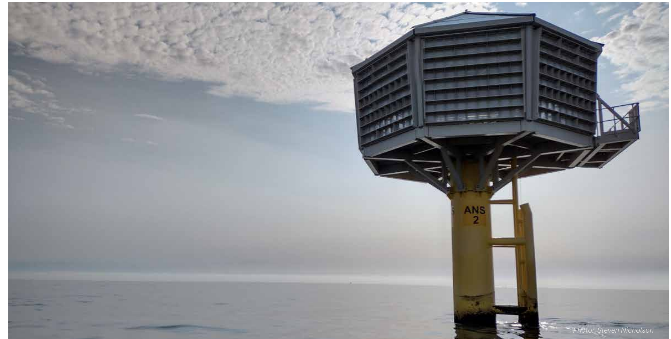
An ANS is an independent marine structure comprising of an octagonal topside with individual nesting spaces supported above the water on a single monopile. Each ANS has capacity for around 500 nesting spaces spread across eight rows of ledges per nesting face.
